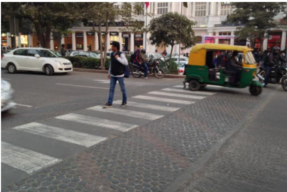
Raised pedestrian crossing
